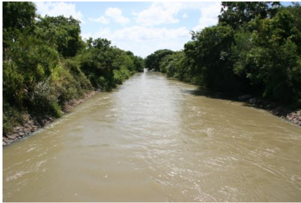
Figure 9. A modern feeder canal with paved embankments on both side and steep gradient.
