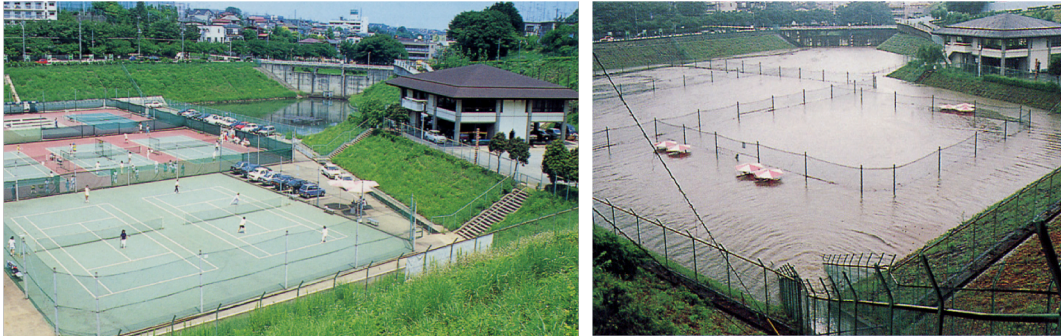
Figure 5. Use of urban facilities and temporary flood control measures (courtesy: Association for Rainfall Storage and Infiltration Facilities (ARSIT))
